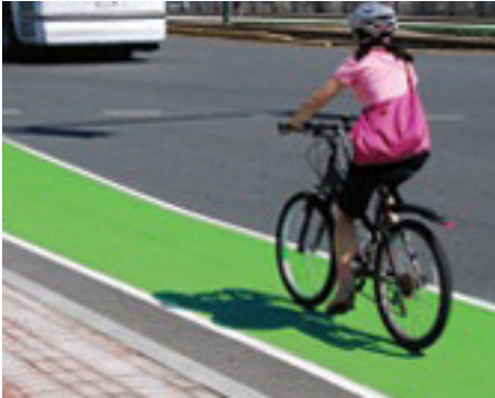
Example of Epoxy Bike Coating on Asphalt
